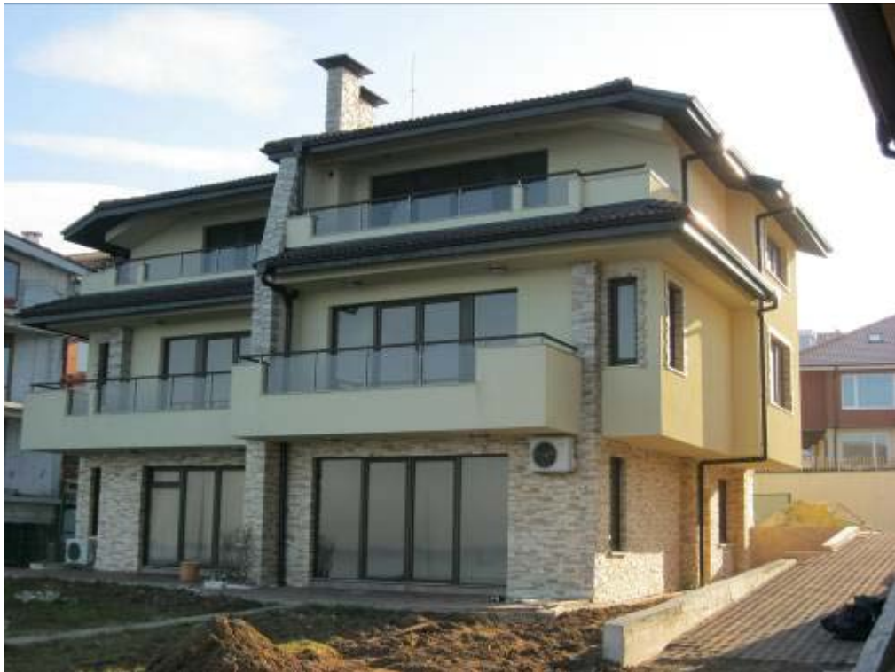
Complex “Orfey DV” – Budjaka area, town of Sozopol
