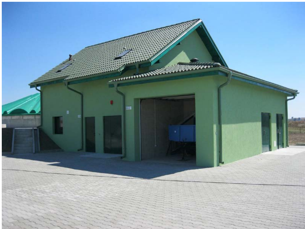
Waste Water Treatment Plant Tenevo – Yambol Municipality
