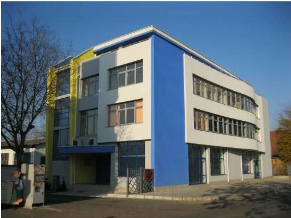
Administrative building “Alex” – Burgas
